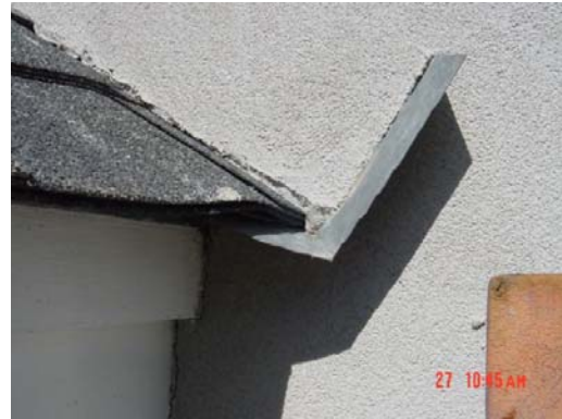
Detail Photo #2 -- Kickout flashing is present. Seal all kickouts.
