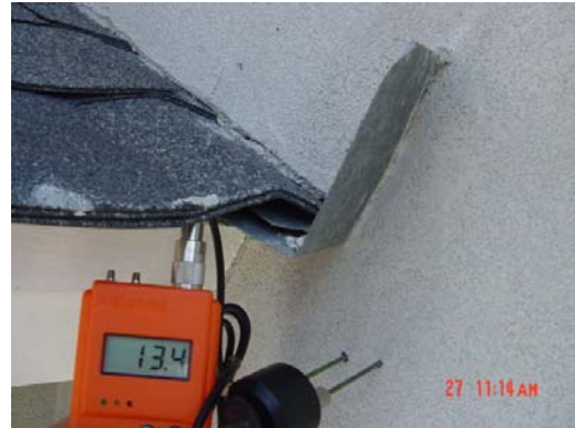
Detail Photo #8 -- Kickout flashing is present. Seal all kickouts.
