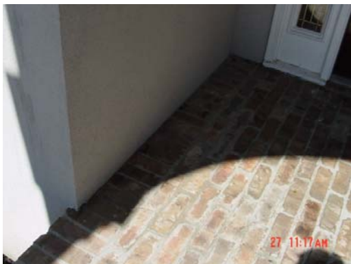
Detail Photo #11 -- Porch Floor Termination.
