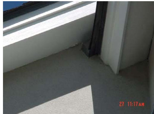
Detail Photo #10 -- Kickout flashing is present. Seal all kickouts.
